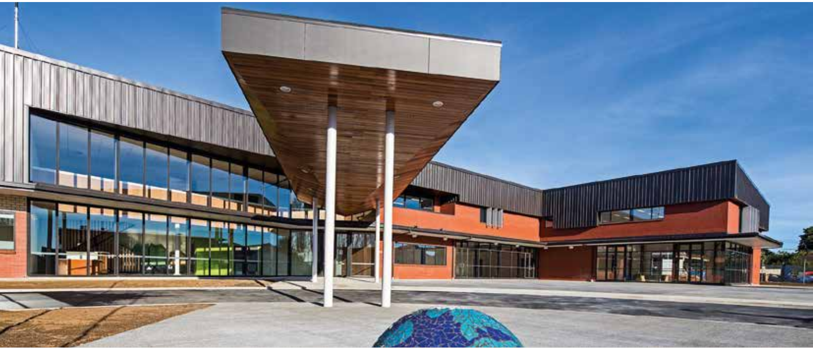
Finished project: Mangere Refugee Resettlement Centre.
